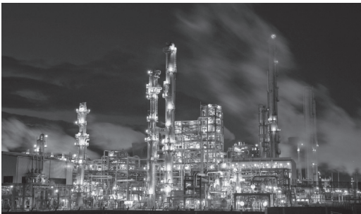
□ Reliance Jamnagar Complex
